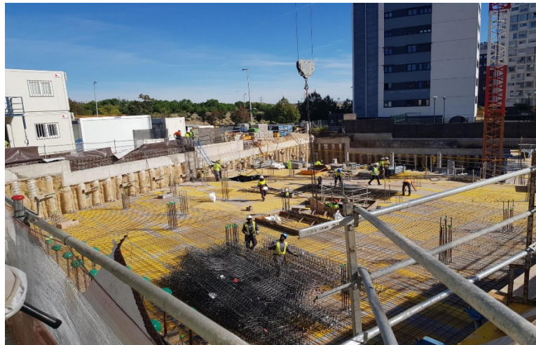
Figure 2: Structure phase in construction work (Madrid).
